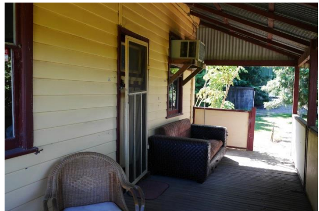
Figure 3 Corrugated metal verandah on northern façade, supported by timber posts, with hardwood flooring.
