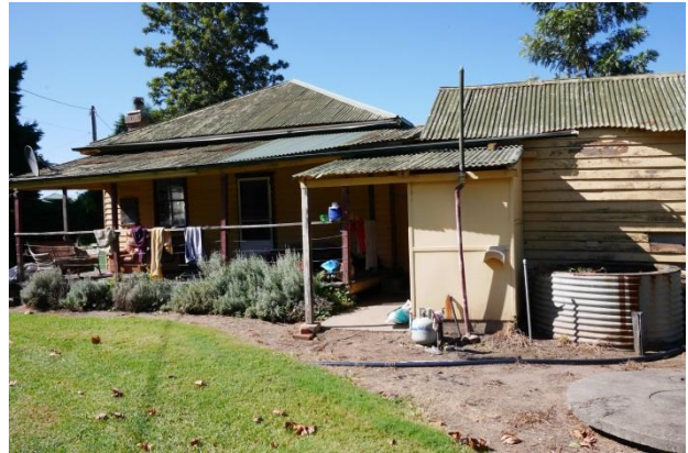
Figure 5 Northern elevation of farm building showing toilet/laundry extension (Source: GML 2016)
