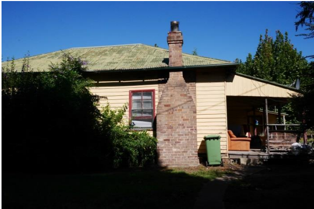
Figure 4 Western elevation of farm building (Source: GML 2016)
