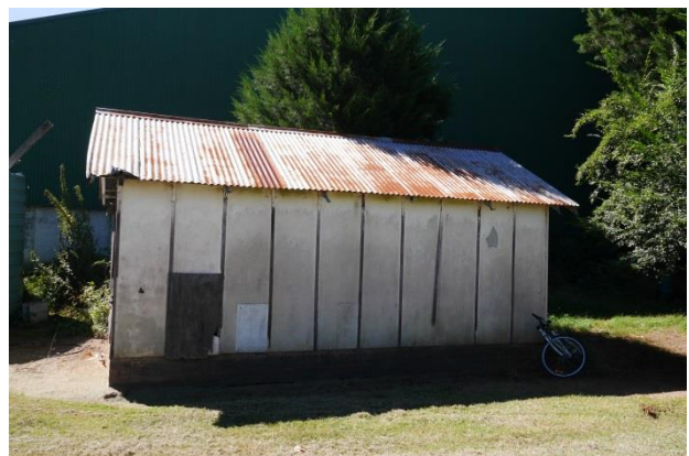
Figure 9 Storage shed (Source: GML 2016)
